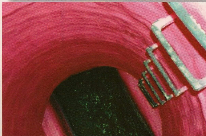
The project resulted in 142 manholes being rehabilitated.
